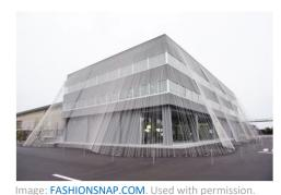
Fa-bo, an office building in Japan, has **carbon-fibre cables** connecting the roof of the building and the ground. If an earthquake hits, the cables stretch and pull in the opposite direction to the shaking, keeping the building standing.
