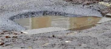
At higher speed, hitting a deep pothole can cause severe damage and also risks loss of control resulting in impact with other vehicles, the kerb or roadside objects.
