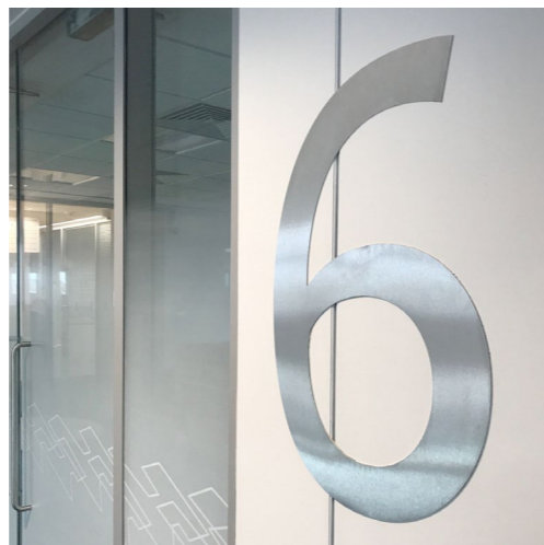
Stainless steel floor numbers applied to walls
